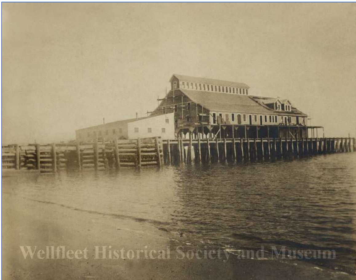
Figure 13 - Chequesset Inn under construction 1902 (© WHSM)
