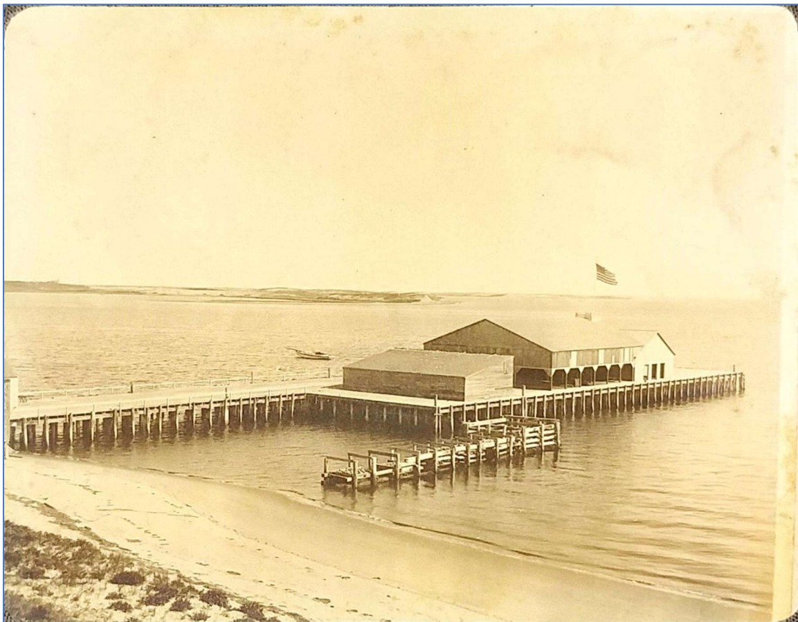
Figure 12 - Mercantile Wharf Company
